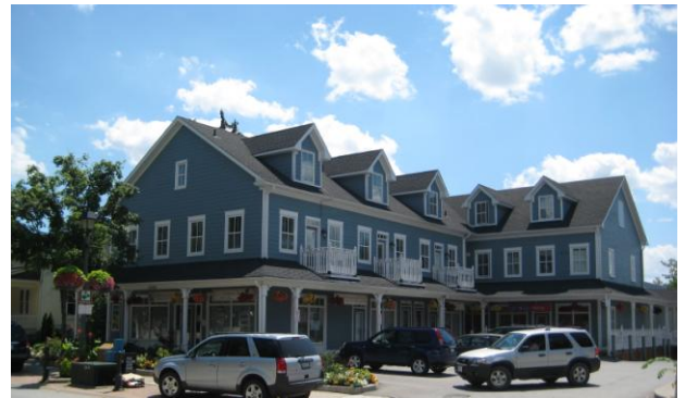
The Post Office Building
